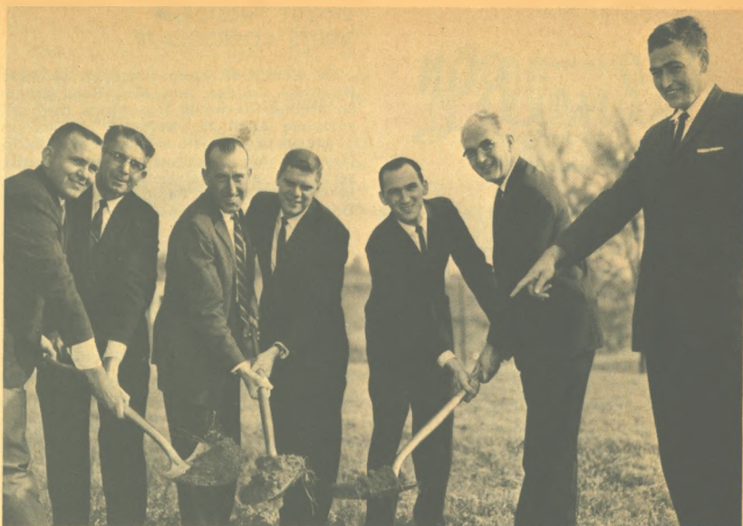
GROWING CHURCH —Laymen and ministers join in breaking ground for the new Estill Springs, Tennessee, church now under construction. From left to right are Glenn Hill, Hobart Hill, and Preston Hill, trustees; Pete Garner, city alderman; Pastor Richard Reed; Rev. Victor E. Gray, superintendent of the East Tennessee District; and Elbert Brown, trustee.
