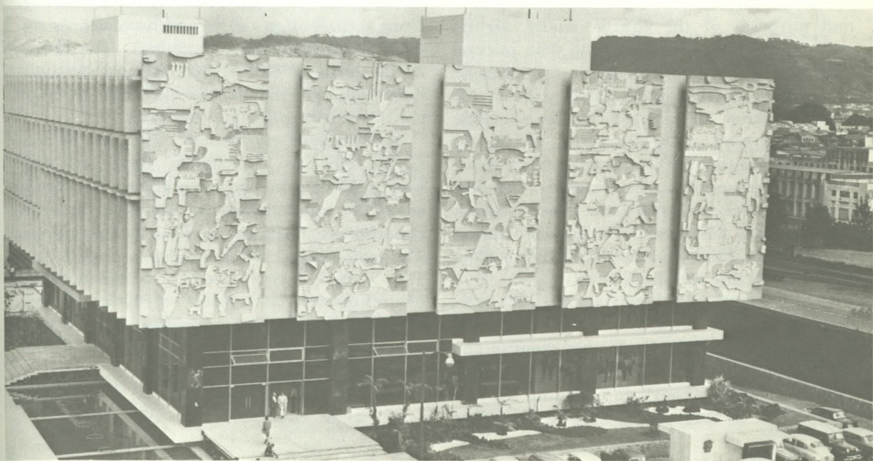
RECENTLY completed National Bank in Guatemala City
