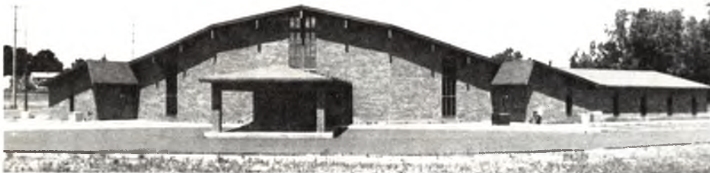
The Westland, Mich., church recently dedicated their new facility. Situated on a nine-acre tract of land the building has 11,113 sq. ft. of floor space. The sanctuary will seat 300 people, including the choir. There are 12 Sunday School classrooms, a fellowship hall that will seat about 200 people, a baptistry, and office rooms. General Superintendent Charles H. Strickland delivered the dedicatory message, and District Superintendent Marselle Knight offered the dedicatory prayer. Other guests included former pastors, Rev. John Mellish, Jr., and Rev. Alan Dicer. The estimated value of building and property is $750,000. Pastor Stephen R. Lowe has served the Westland congregation since 1984.
