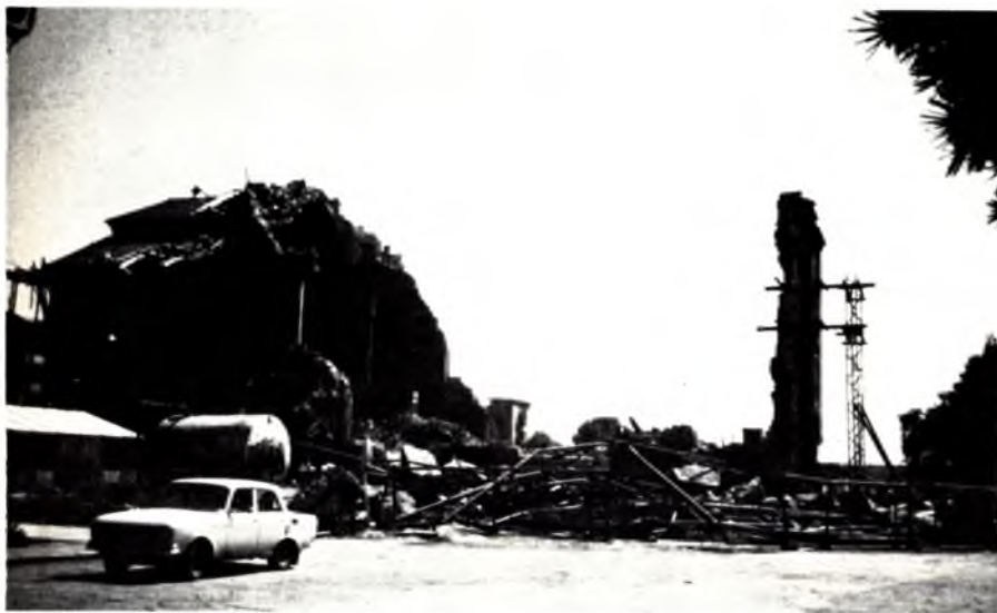
A former church in Leninakan that was destroyed by the 1988 earthquake.
